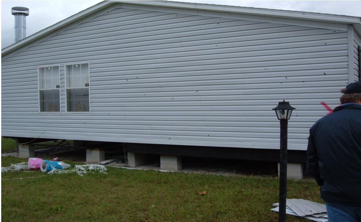
These two mobile homes had the Byrd system installed and only had minor skirting damage.
