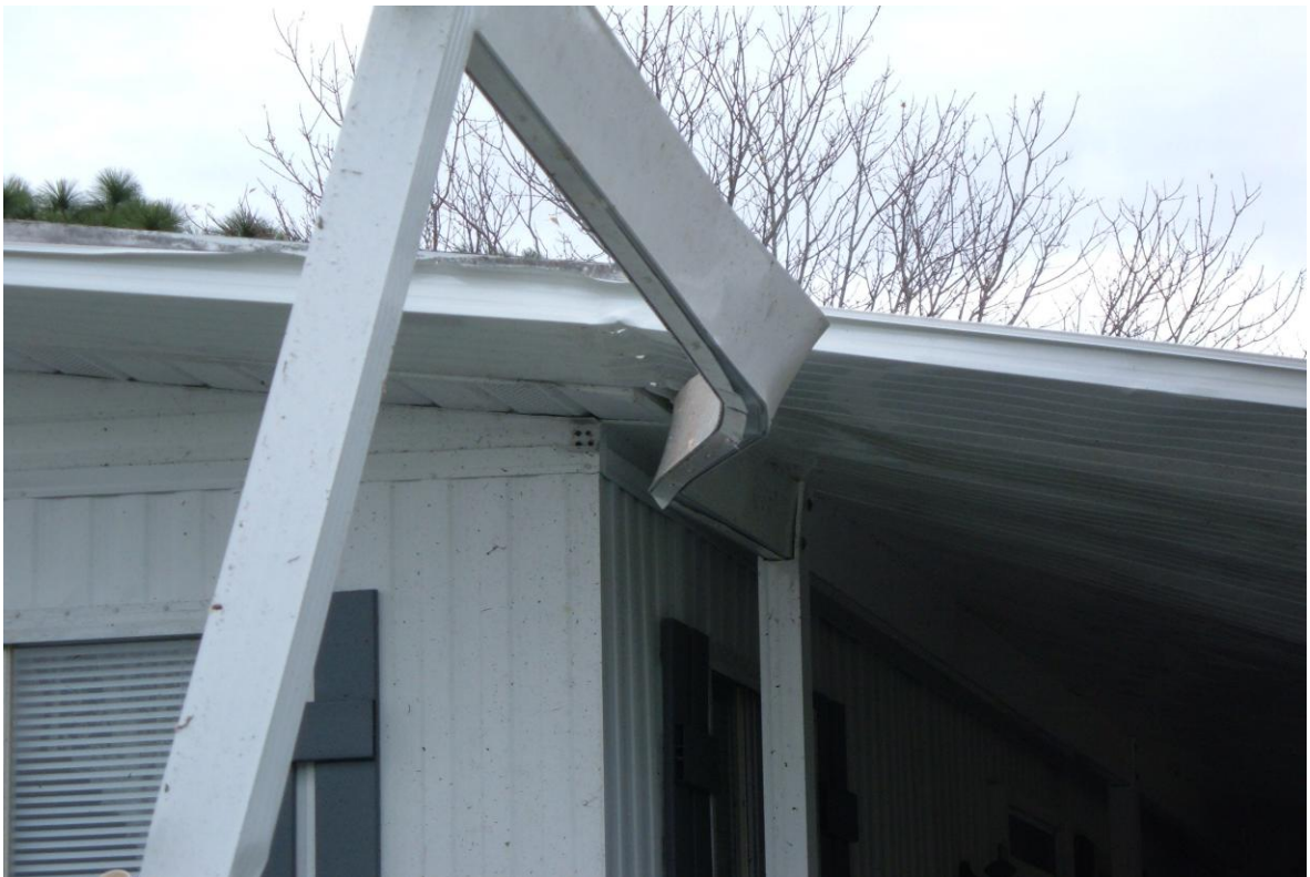
The aluminum attachment to the above home caused the damage to the roof. The picture below is of a home with a fourth wall that prevented the home from being totaled.
