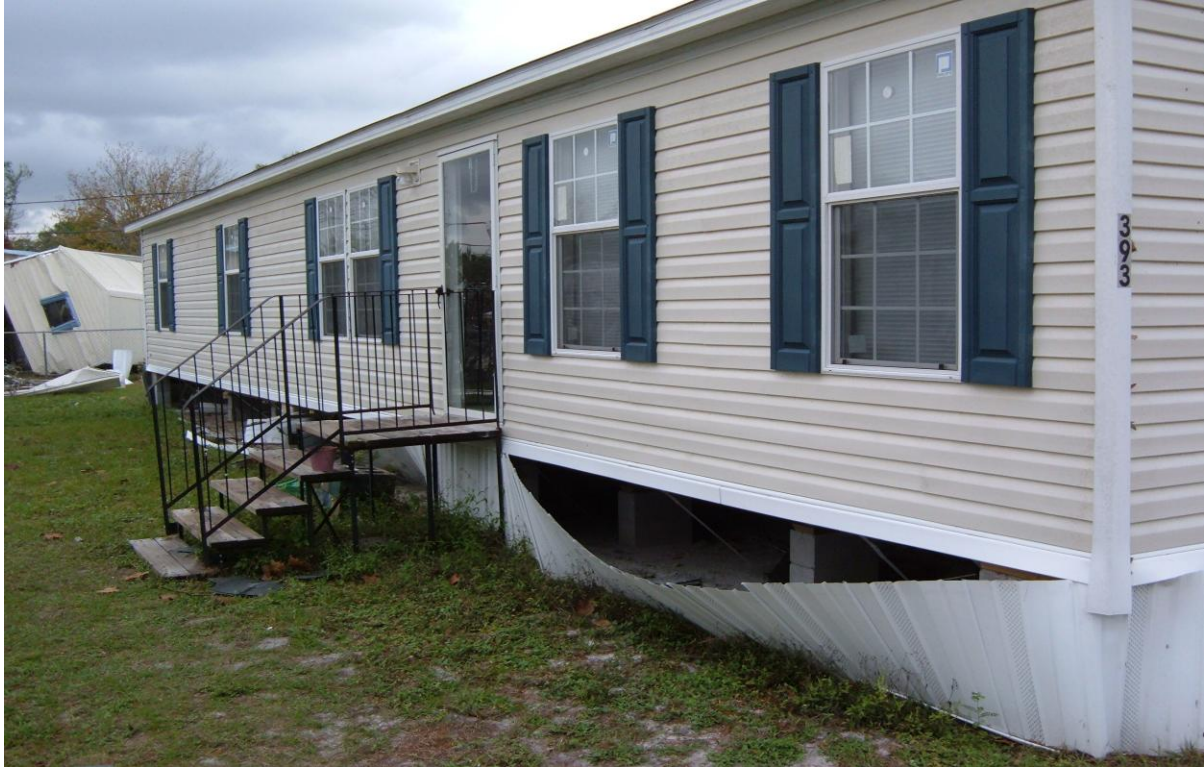
These two mobile homes had the Byrd system installed and only had minor skirting damage.
