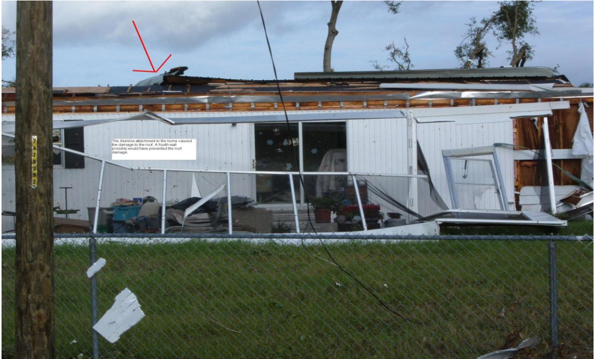
The aluminum attachment to the above home caused the damage to the roof. The picture below is of a home with a fourth wall that prevented the home from being totaled.
