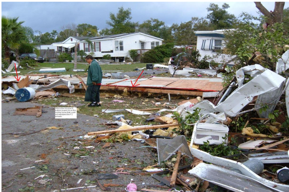
These pictures show the rim-joist rot on the mobile homes that caused the walls to collapse during the F-2 tornado.
