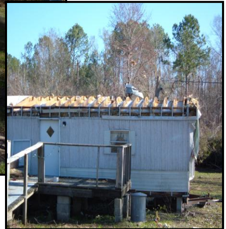
The home moved off its foundation due to rusted anchors, too few anchors and the straps were improperly spliced.
