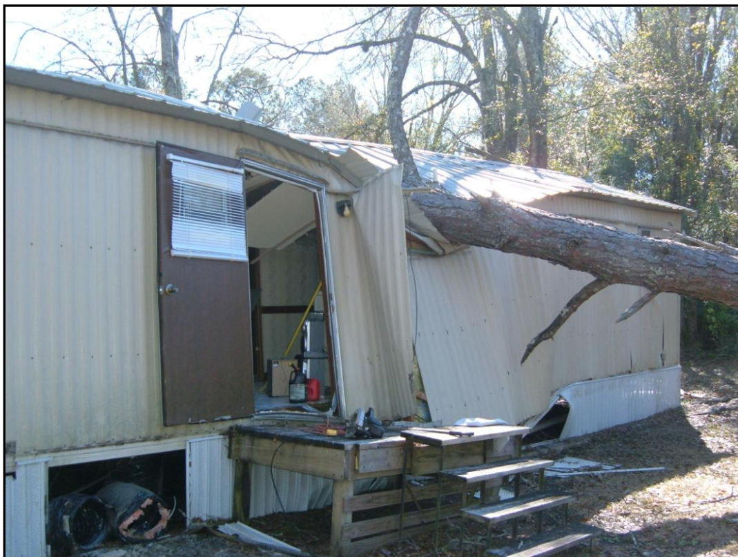
A home severely damaged due to a fallen tree. Front and back view. The home stayed on its foundation.
