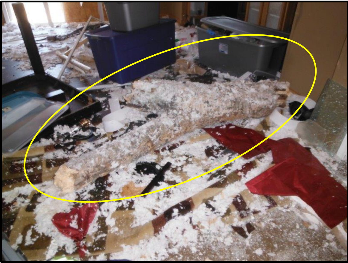
Another hazard – flying debris. This is a very large limb that penetrated the roof of this manufactured home.
