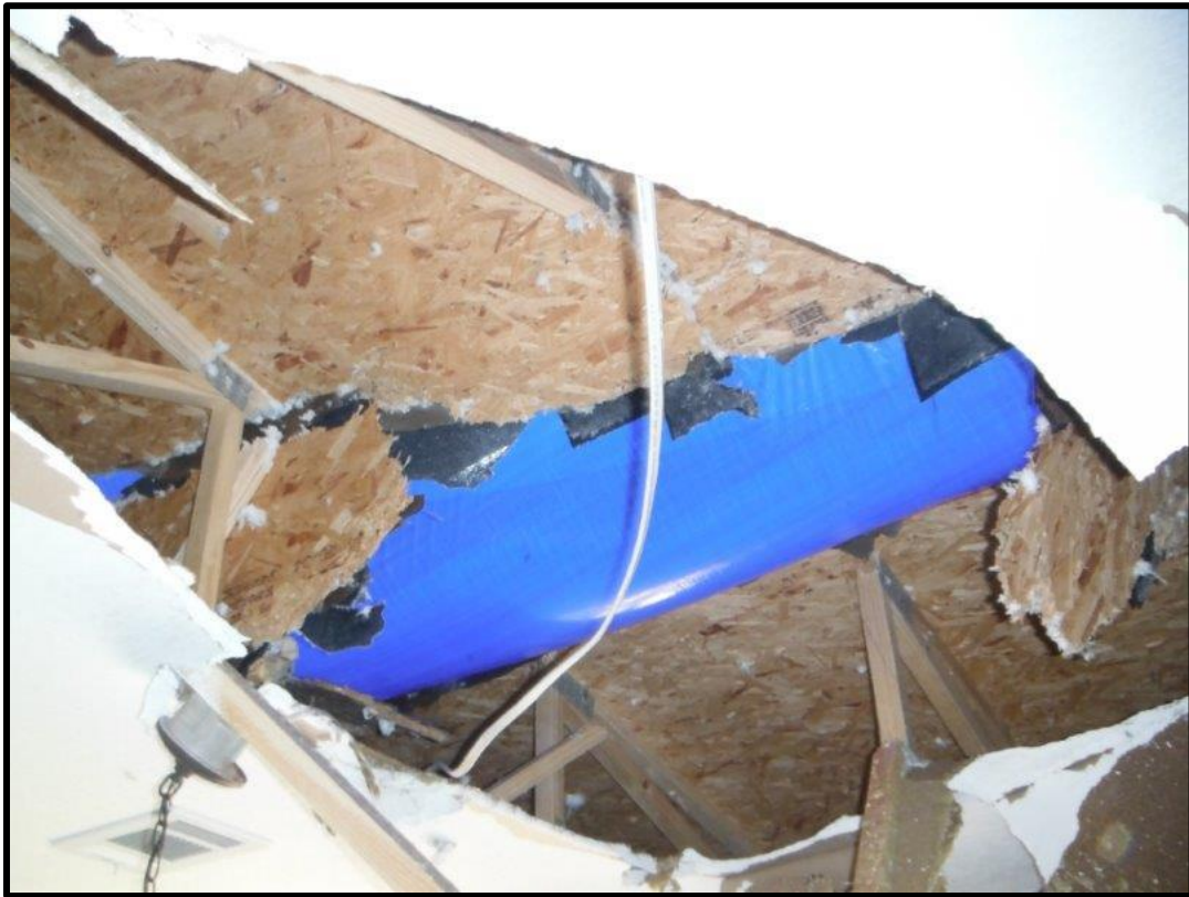
Another hazard – flying debris. This is a very large limb that penetrated the roof of this manufactured home.
